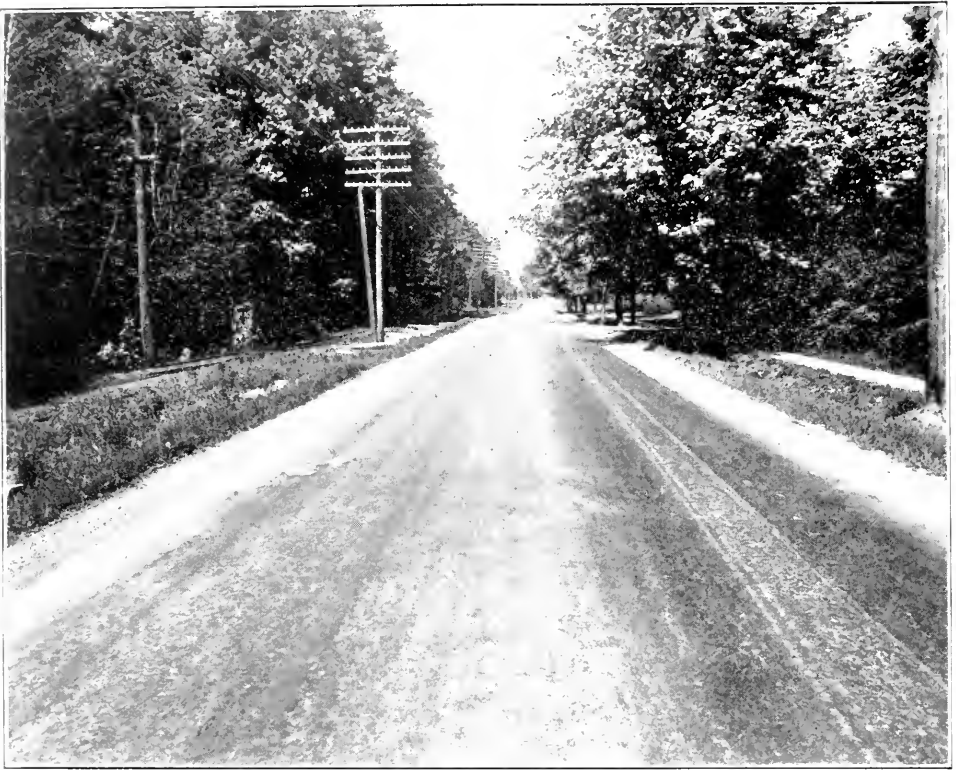
Old bituminous penetration road on the Hamilton-Queenston Highway surface treated in 1927 with 1/8-gallon Heavy Cutback Asphalt and 15 pounds stone chips and coarse sand per square yard.
